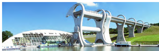
The Falkirk Wheel raises 600 tonnes of water over (115ft) in under 4 minutes, using only 1.5kW energy.
